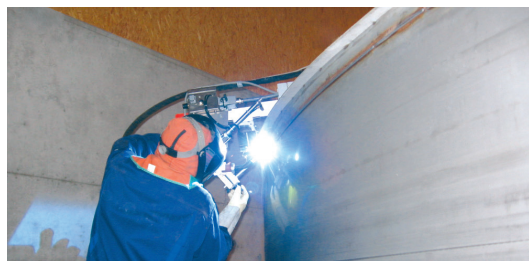
The conical type of roof is welded to the tank jacket.
