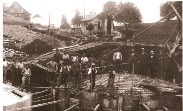
Tank construction in 1926
